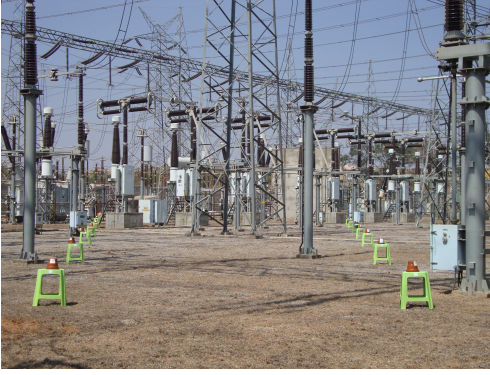
Fig. 3. A view of the 440 KV power distribution yard, showing the layout of equipment; apart from the transmission towers, several transformers and a firewall can be seen at a distance.
