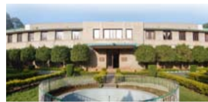
Electrical Communication Engineering (ECE)
