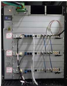
LTE eNB (Base Station)
